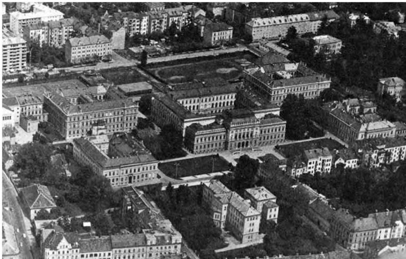
FIGURE 3: The campus of the Karl-Franzens-University Graz – the picture dates from ca. 1960 and shows the campus as it has been set up in the time between 1870 and 1905 in its original status: the eldest building (anatomy and physiology) can be seen in the middle directly in front in a small park), then physics (1876, in front left side) and chemistry (1879, at the right side) between the main building (1895); in the background at left the building for theoretical medicine disciplines and at right the building for natural sciences (inside the faculty of philosophy). The buildings for physics and for chemistry at the time of their construction were worldwide famous – physics partially was built without iron in behalf of special experiments, first professor working there was Ludwig Boltzmann. – Today this campus is still the nucleus of the enlarged university. The clinics of both universities were and are outside; in Graz a new large hospital area with a lot of buildings was opened in 1912. Archive of the Karl-Franzens-University of Graz.
